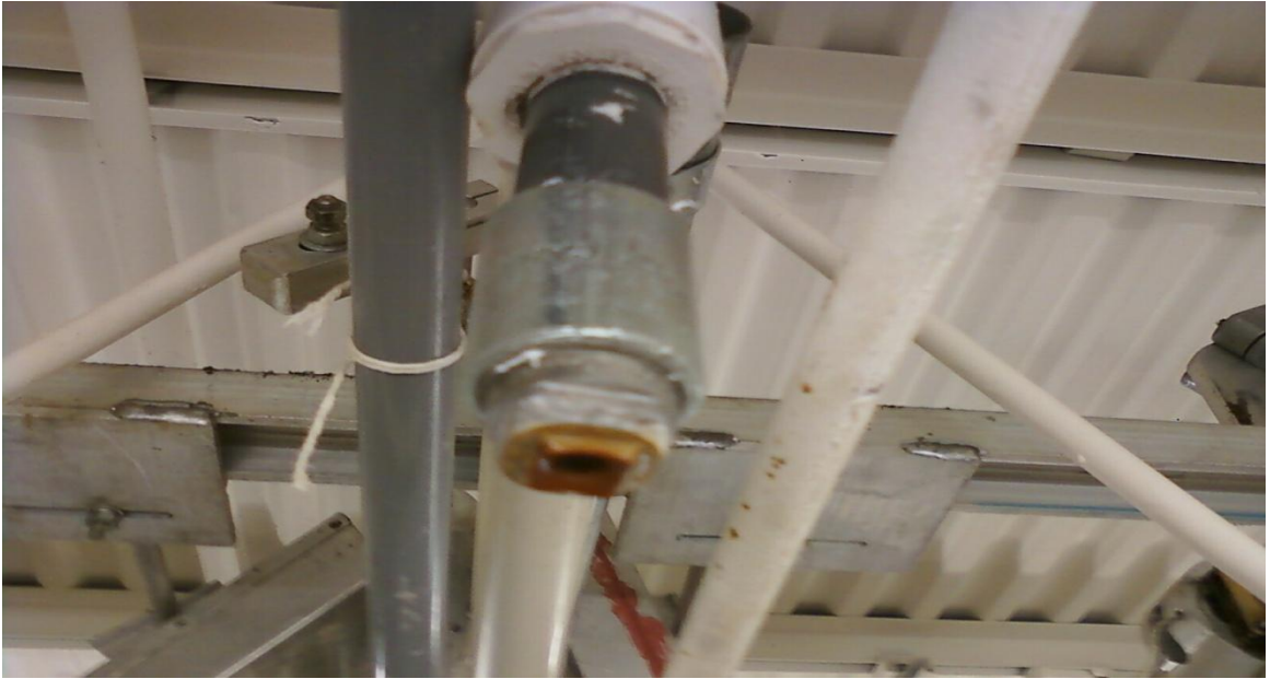
Figure 2.2: An example of a square nozzle-type rainfall simulator of the Agricultural Engineering Building of the University of Missouri-Columbia.
